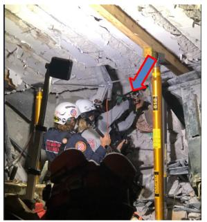
Image 4: Search camera used to view behind the slab.
